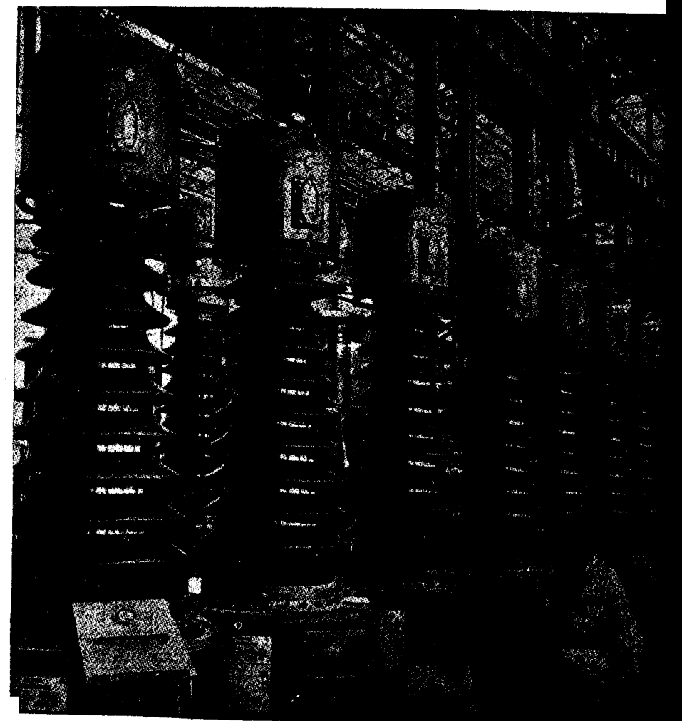
BELOW : A long line of 132 KV single phase transformers manufactured at the factory.
