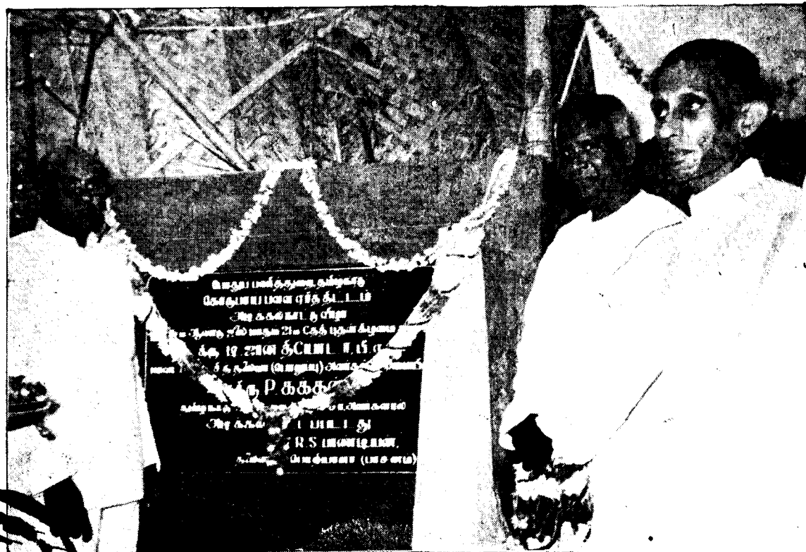
FOUNDATION TABLET FOR GODUBAIPALLAM SCHEME LAID ON 21ST JULY 1966.
