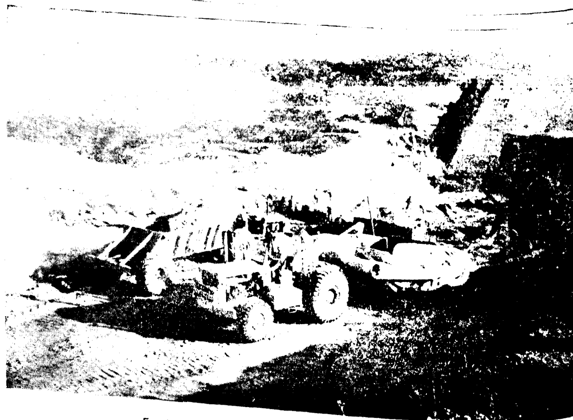
Earth movers in action at the Sholayar Dam site.
