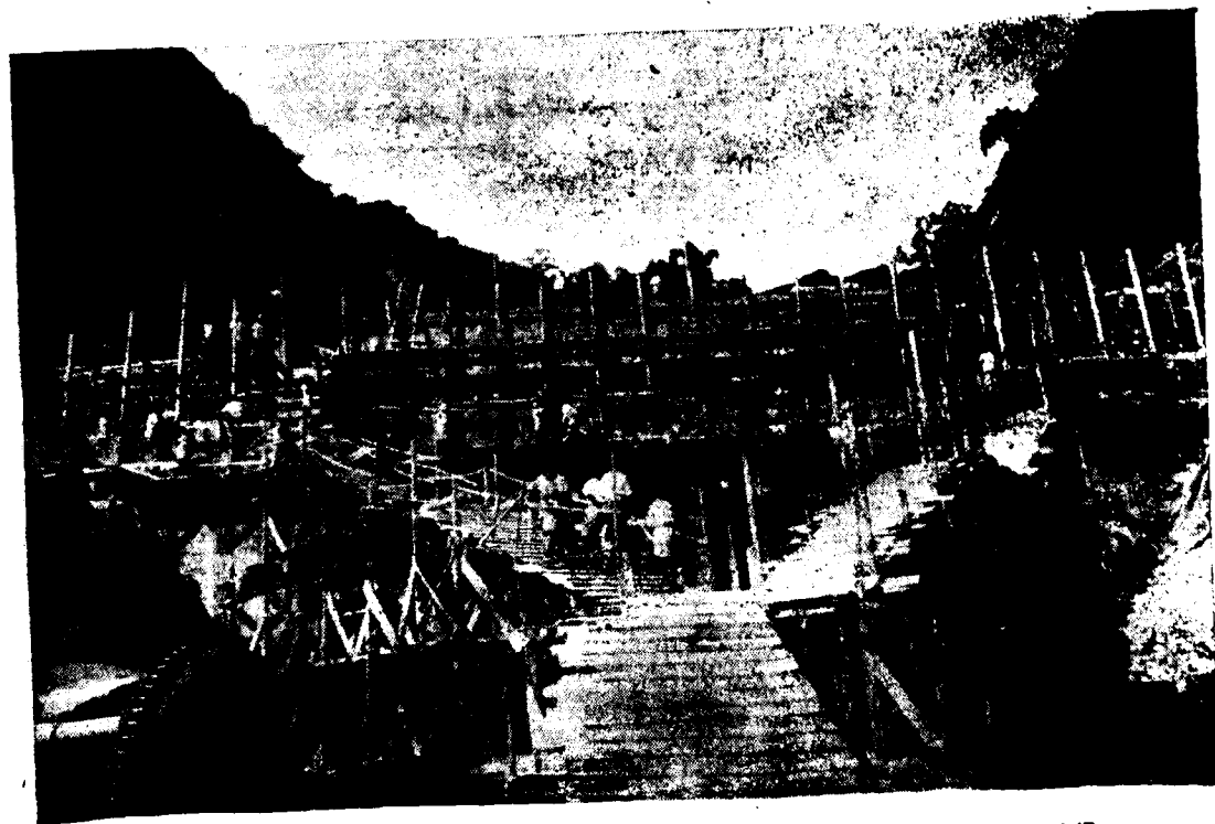
Contour canal—Direct view of aqueduct across Chinnar near mile 9/7.
