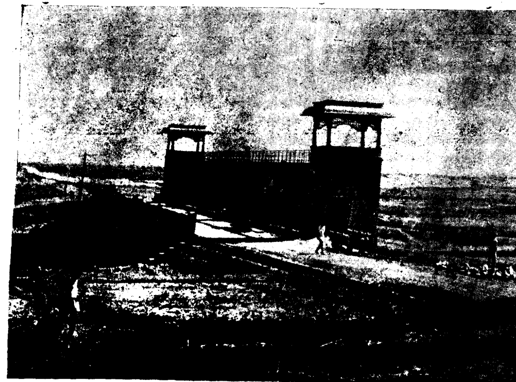
View of surplus Regulator - Thirumurthi Dam.
