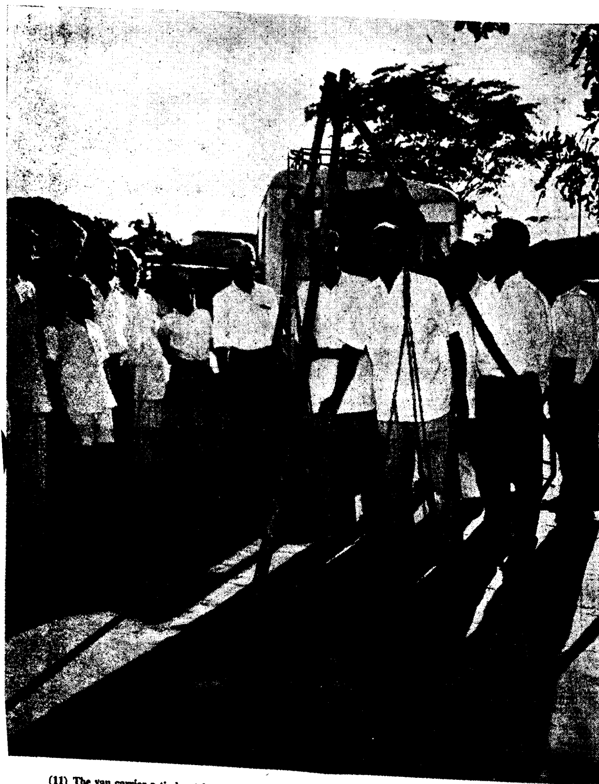
(11) The van carries a timber tripod which can be used for the verification of heavy capacity beam scales. For verification of these beam scales, it is necessary to set up this tripod at a suitable place outside the van. Test weights and working standard weights are used for checking up the accuracy of the beam.
