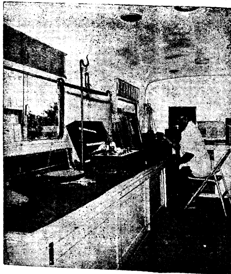
(3) This shows the left hand side of the laboratory portion of the van. The Inspector of Weights and Measures is seen getting ready to verify cast iron weights. The arrangements for the verification of small beam scale, and the working standard length measure can also be seen in the foreground. The sliding shelves can accommodate all the equipment, stationery and publicity literature etc.
