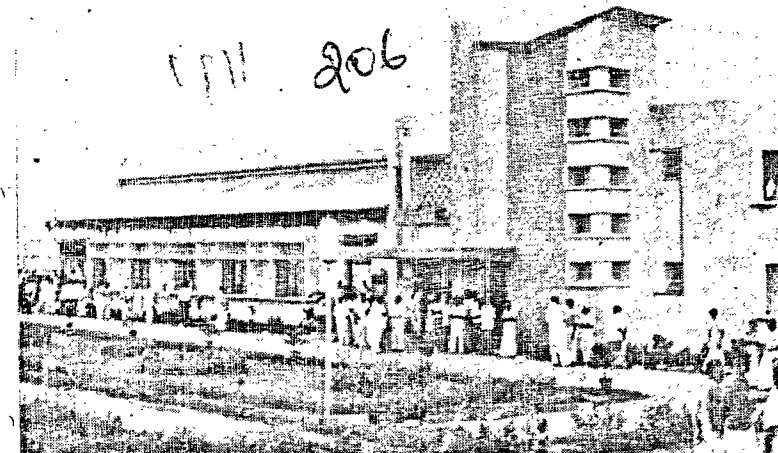
A view of the General Purpose Workshop which was inaugurated by the Chief Minister of Madras on 11th October 1965.
