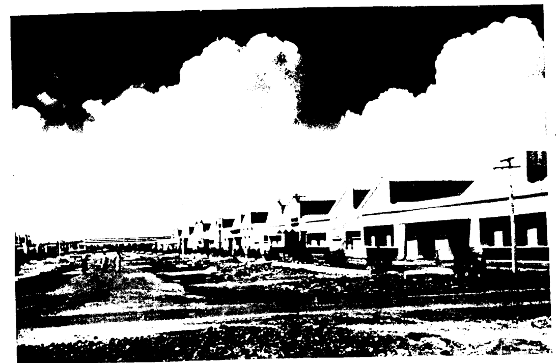
An impressive row of ready built factories in Ambattur Industrial Area.
