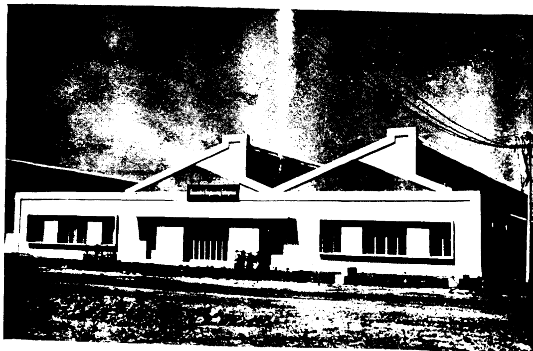
An exterior view of an 'A' type unit in Ambattur Industrial Area.
