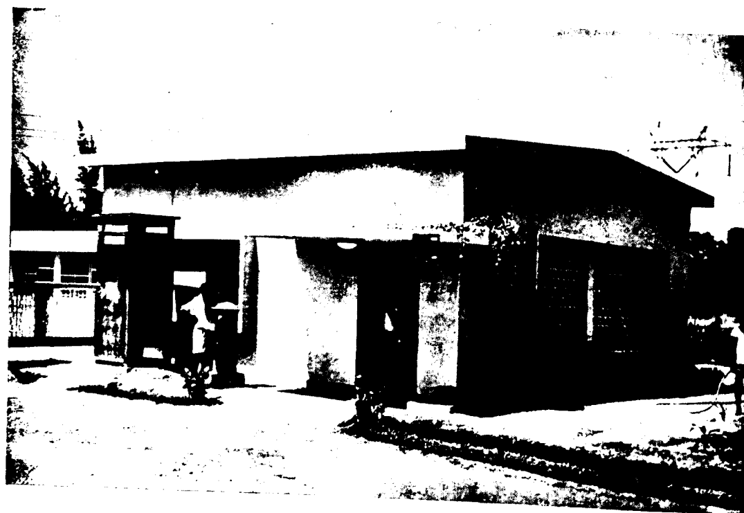
The Post Office building.
