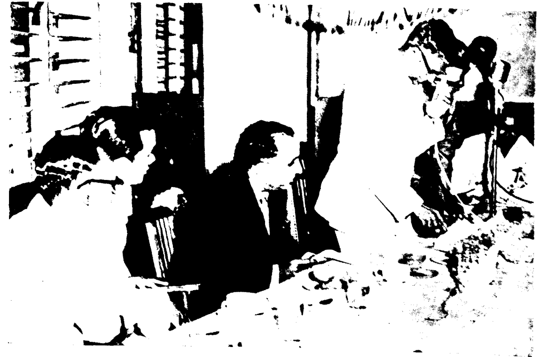
An automatic telephone exchange was installed at the Ambattur Industrial Estate on 12th Feb. '64. Sri R. Venkataraman, Minister for Industries, who inaugurated the exchange is seen dialing the new telephone. Sri T. N. Lakshminarayanan, Secretary, Industries, Labour & Co-operation Department, is seen third from left.
