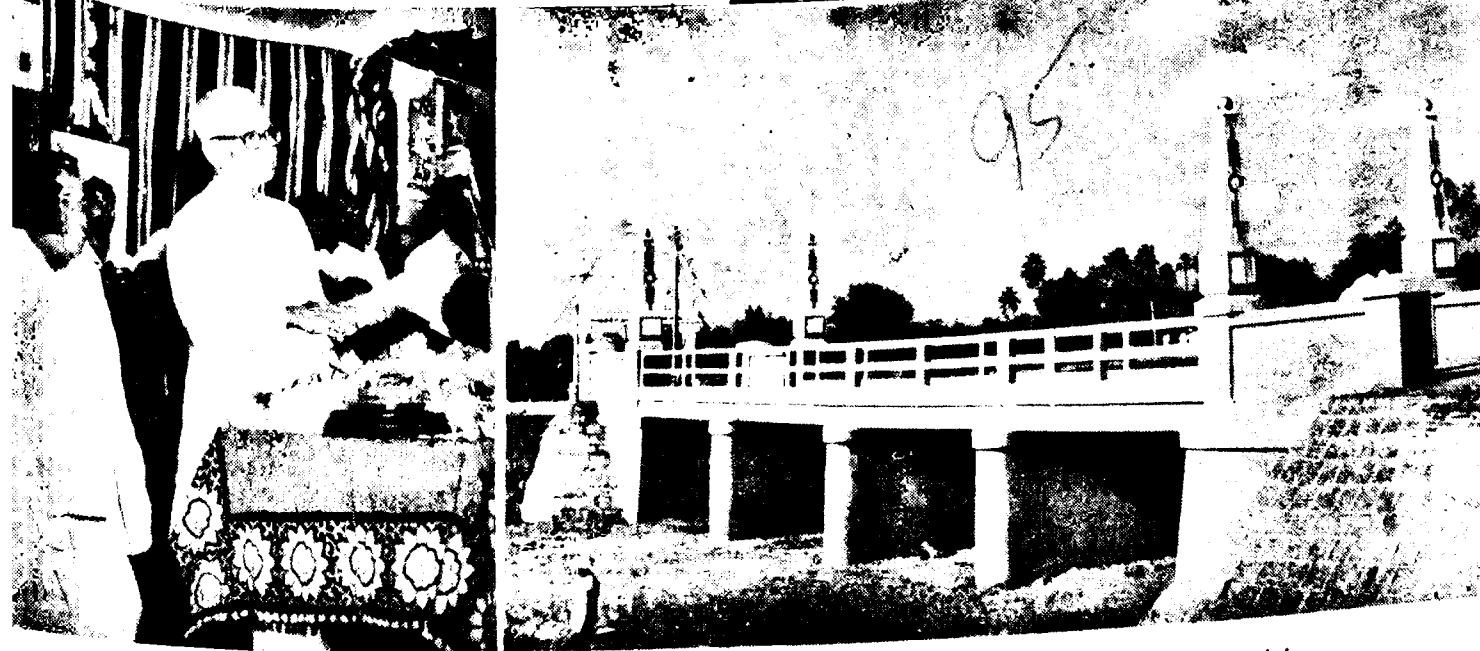
Sri M. Bhaktavatsalam, Chief Minister, declared open the bridge at Tirupayayathamkudi village at Tirumarugal block in Thanjavur district on 29th March 1964. Sri S. M. A. Majid, Minister for Municipal Administration, presided.
