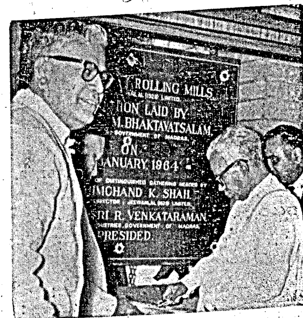
Sri M. Bhaktavatsalam, Chief Minister, laid the foundation stone for Aluminium Rolling Mills of Jeewanlal Company on 26th January 1964. Sri R. Venkataraman, Minister for Industries, presided.
