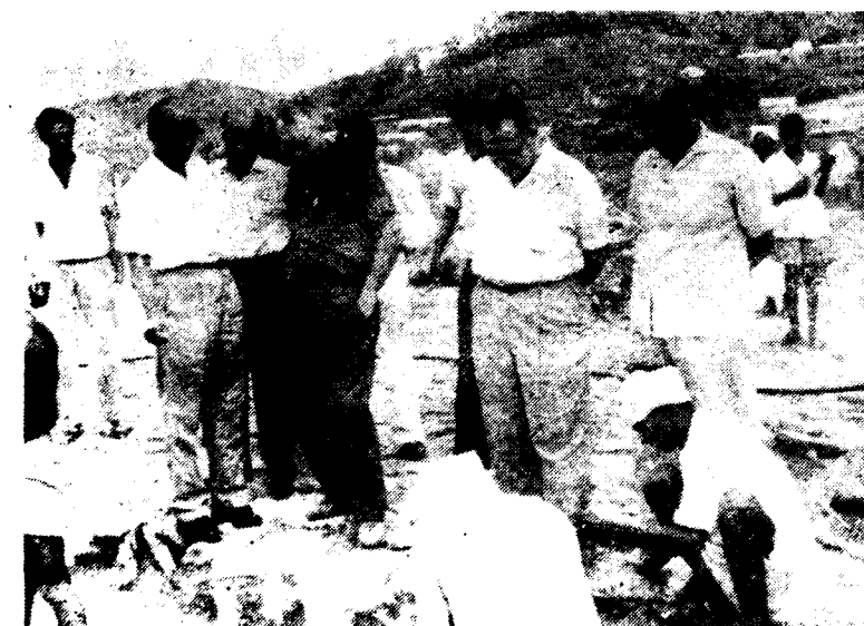
World Bank Team inspecting masonry work in progress at Sholigar Dam.
