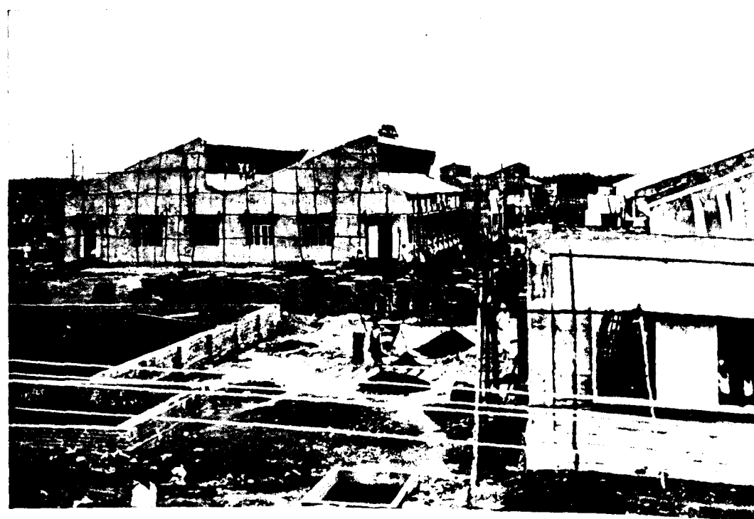
Factory sheds under construction.
