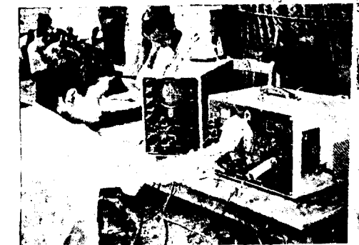
7. Electronic Instruments used for recording dynamic strains.
