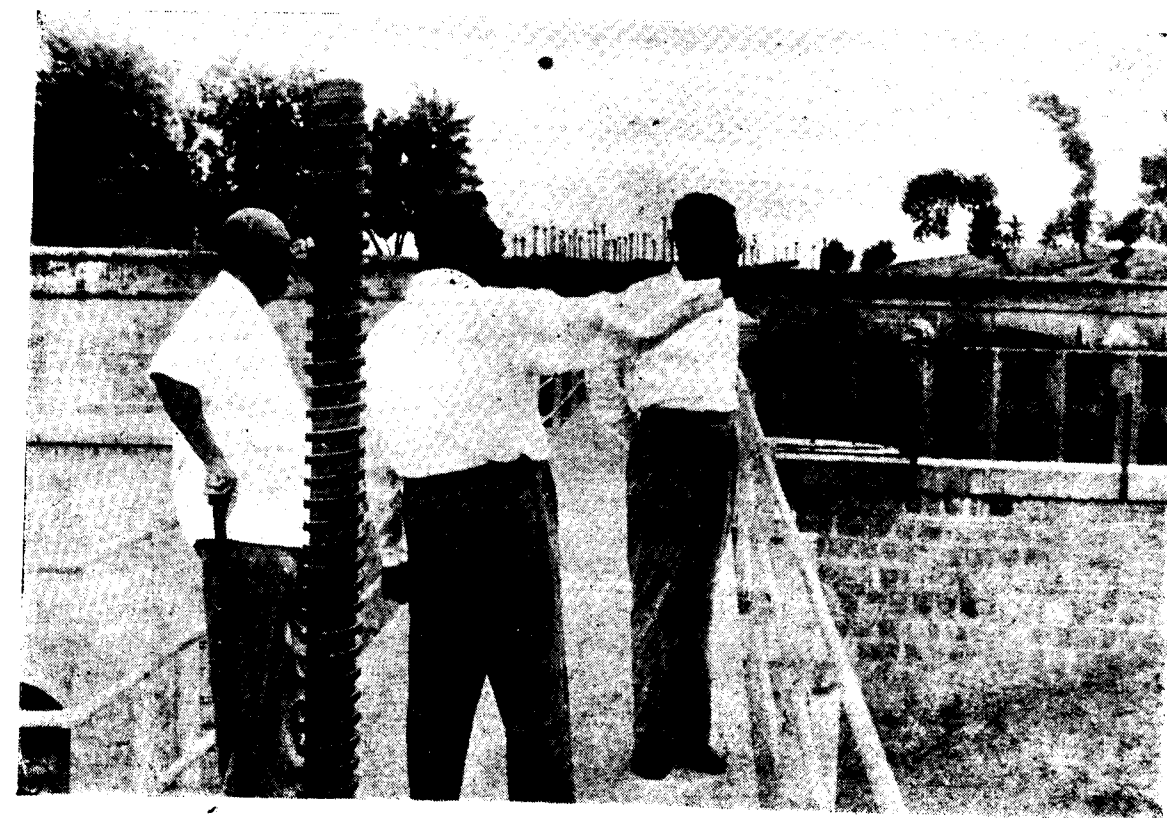
The member being shown the improvements to the branching of the two arms of the Palar River leading to the head sluices on either flank.
