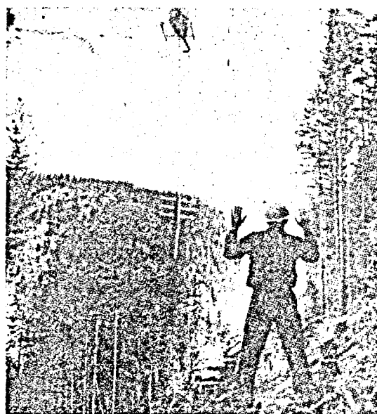
Ground crewman has a hard time maintaining his equilibrium on steep mountain slope as he directs helicopter pilot during installation of telephone poles
