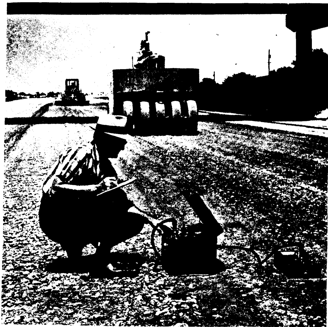
Data for the contractor without waiting. A Texas engineer takes a "reading" on a base course with the nuclear device which radiates gamma rays and fast neutrons to determine density and moisture content.
