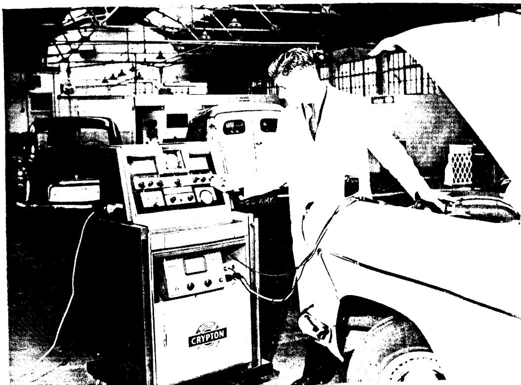
A new electronic tester for testing automobiles. (See article on facing page.)
