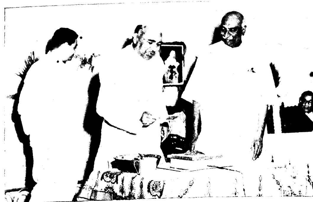
Sri Jagjivan Ram, Union Minister for Transport and Communications, laid the foundation stone for the Hindustan Teleprinters Factory in Madras on July 10, 1962. Sri K. Kamaraj, Chief Minister of Madras, presided over the function. Sri B. S. Rau, Managing Director of the Factory, is on the left.
