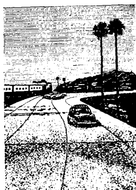
Concrete Road near Madurai
