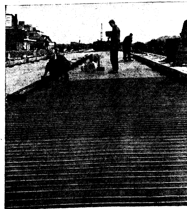
HAMMERSMITH FLYOVER is a vital half-mile section of London's western highway. BICC heating cables were installed to eliminate ice formation.
