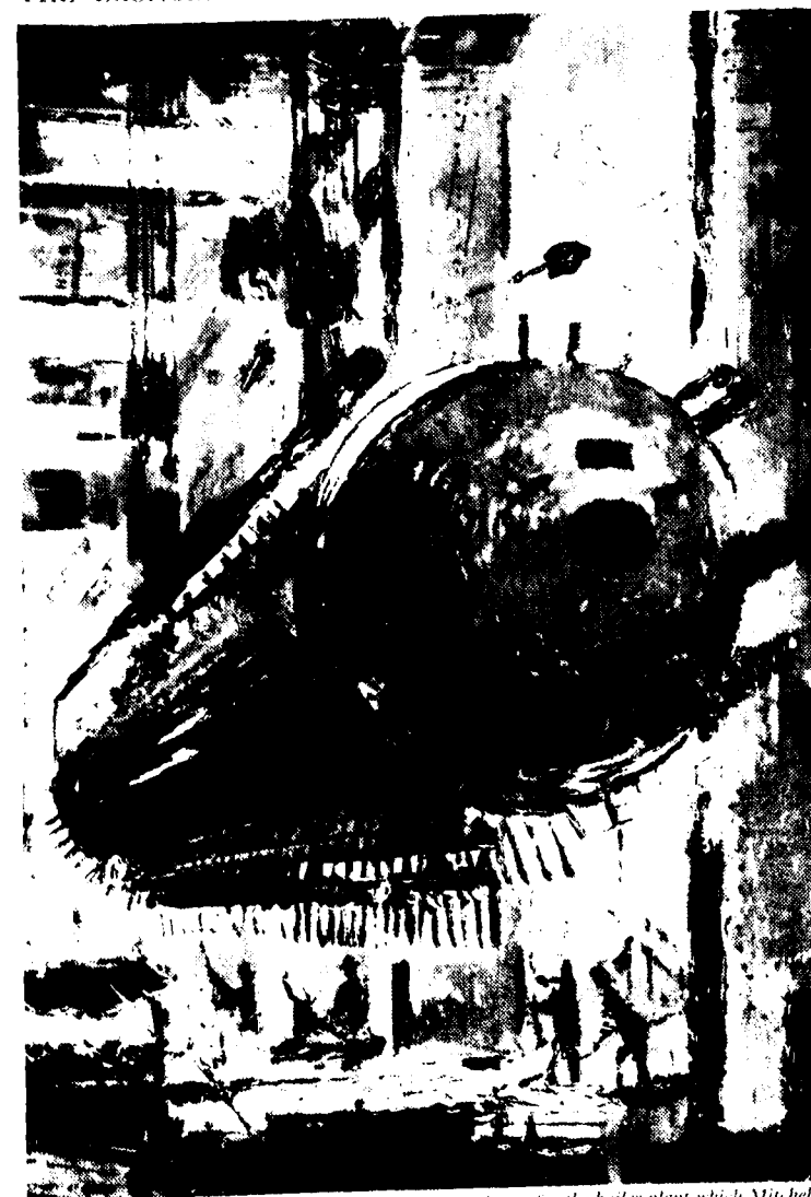
One of the main steam drums for the boiler plant which Mitchell's have installed at Komati power station, Eastern Transvaal.
