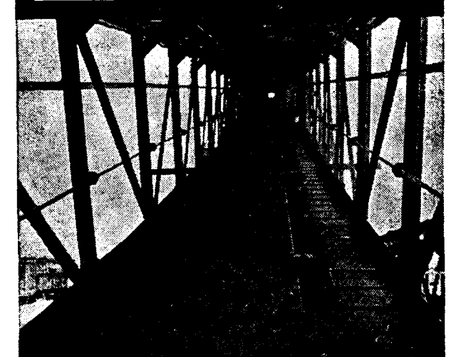
A Dunlop conveyor belt spliced at site and fitted on one of the Simon-Carves conveyors at Durgapur. (Photos: Courtesy ISCON)
