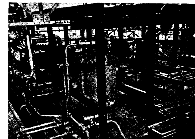
Battery of Type 1 spiral heat exchangers for heat recovery between "new" and "old" sodium aluminate liquors, in a British alumina works
