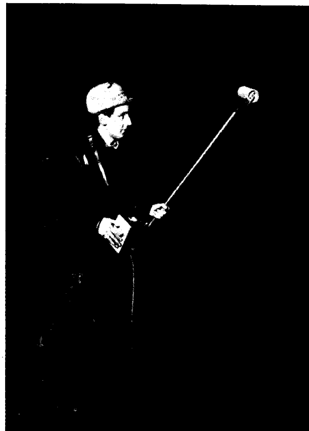
An Inspector checks for continuity of the coating employing a fail-safe wet sponge holiday detector.
