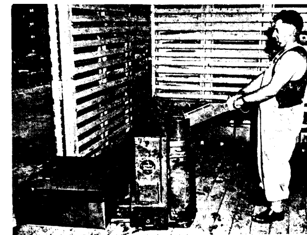
The Transloader model POEP 2 is ideal for operating in confined spaces. A special version designed for handling packs of tinplate is seen here being used to unload railway waggons.
