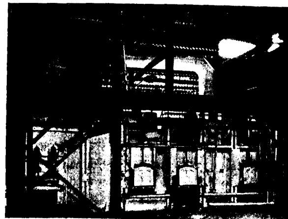
A general view of the side of the furnace, showing the recuperator (top left) and the combustion air duct (top centre) from the recuperator to the air registers
