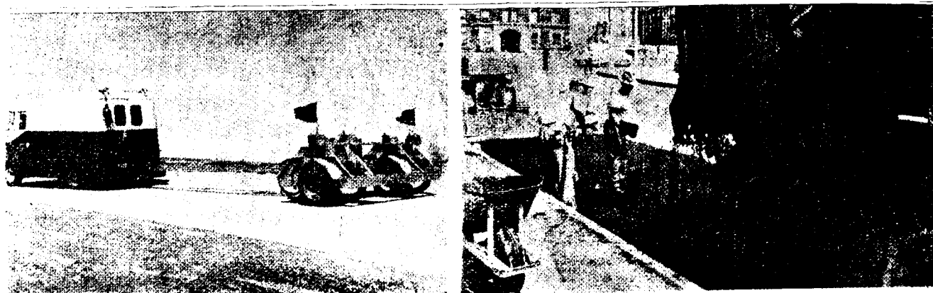
LEFT: Instrument used in American Association of State Highway Officials' Road Test, measures and records roughness of pavements in the wheel paths of the vehicles. RIGHT: Asphalt concrete, dumped from hot mix truck, for resurfacing bus stop on George Washington Bridge.
