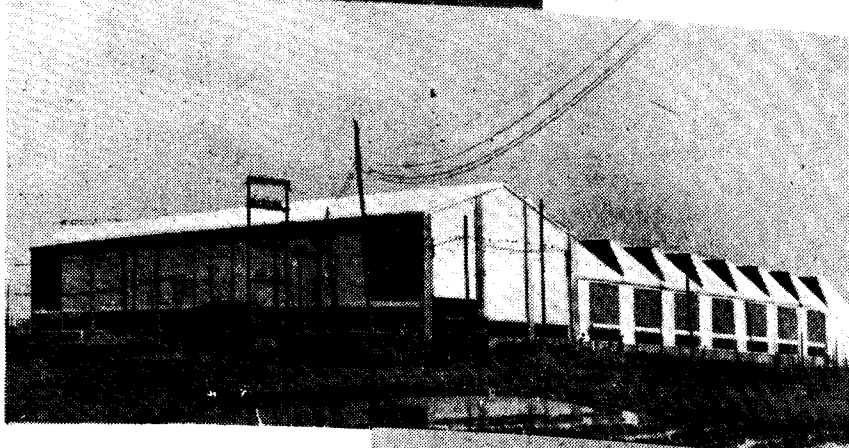
A view of the building for the installation workshop of the Foundry Forge Project, Ranchi, intended for repairs and overhauling of metallurgical and foundry equipment.
