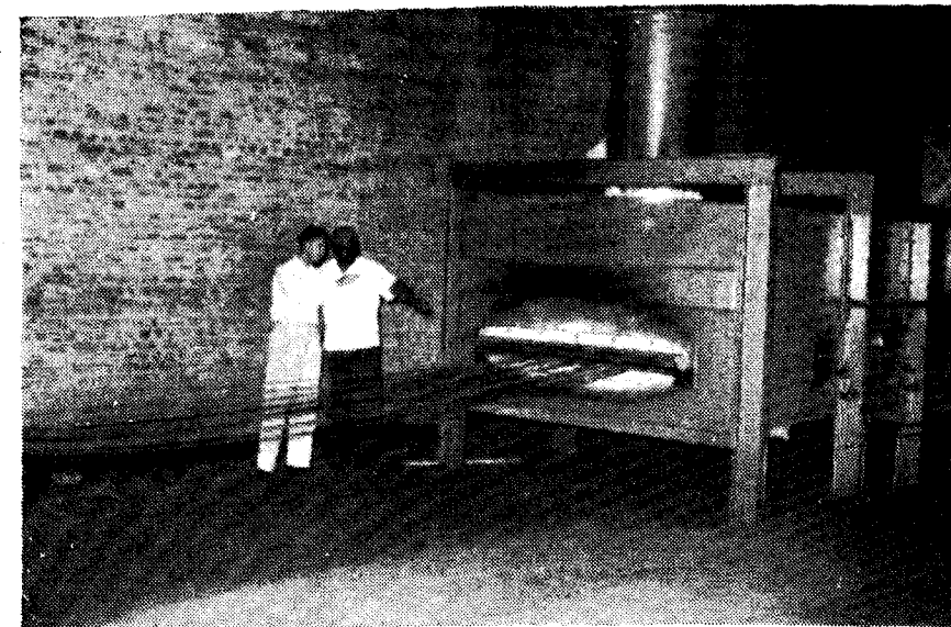
A view of the Normalizing Furnace (Kerosene)
