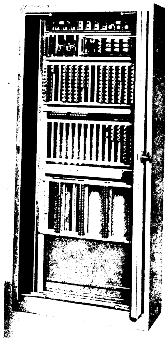
Fig. 1. Typical Remote Control Selector Equipment for Control Centre.
