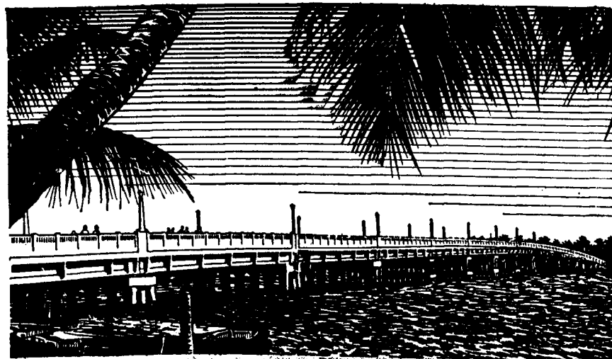
Prestressed concrete bridge on the Bombay-Cape Comorin Road at Aror
