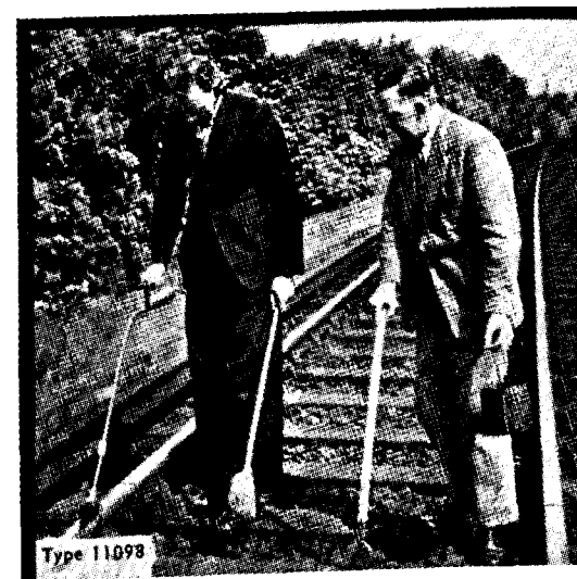
Fig. 6. The DAWE AUDIGAUGE, ultrasonic rail flaw detector, for detecting cracks and other defects in rails and rail joints. The transistorised model gives both visible and audible indication. Weight 5 lbs.
