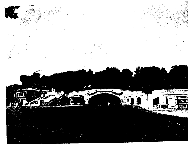
Western Motorway—Paris Access Tunnel
