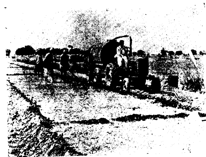
Photograph of experimental asphalt road over soil cement base in Mile No. 46/0 to 47/0 on section Jagudan Mehsana of Ahmedabad-Kalol-Mehsana-Sidhpur Road (S.H.)
