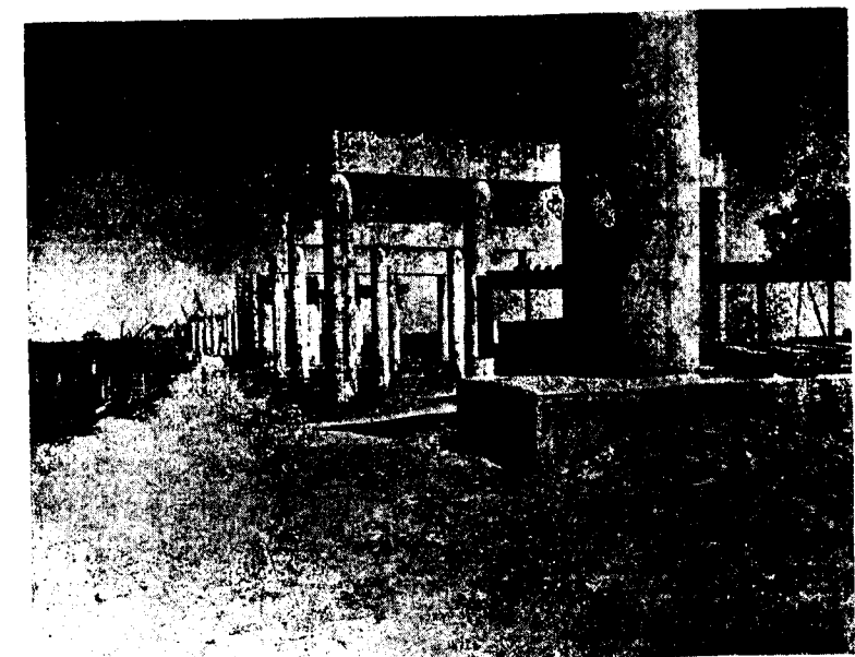
A scene during the building of the Birmingham to Preston motorway, M. 6, in Britain. This picture shows the massive 80 feet high reinforced concrete portal frame piers. They will carry the 28-ton approach span girders of the superstructure for the one and a quarter mile long Thelwall Viaduct. This viaduct will carry the motorway over the Manchester Ship Canal and the River Mersey
