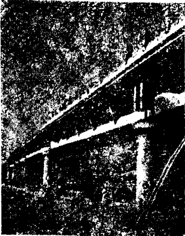
Girders in position
