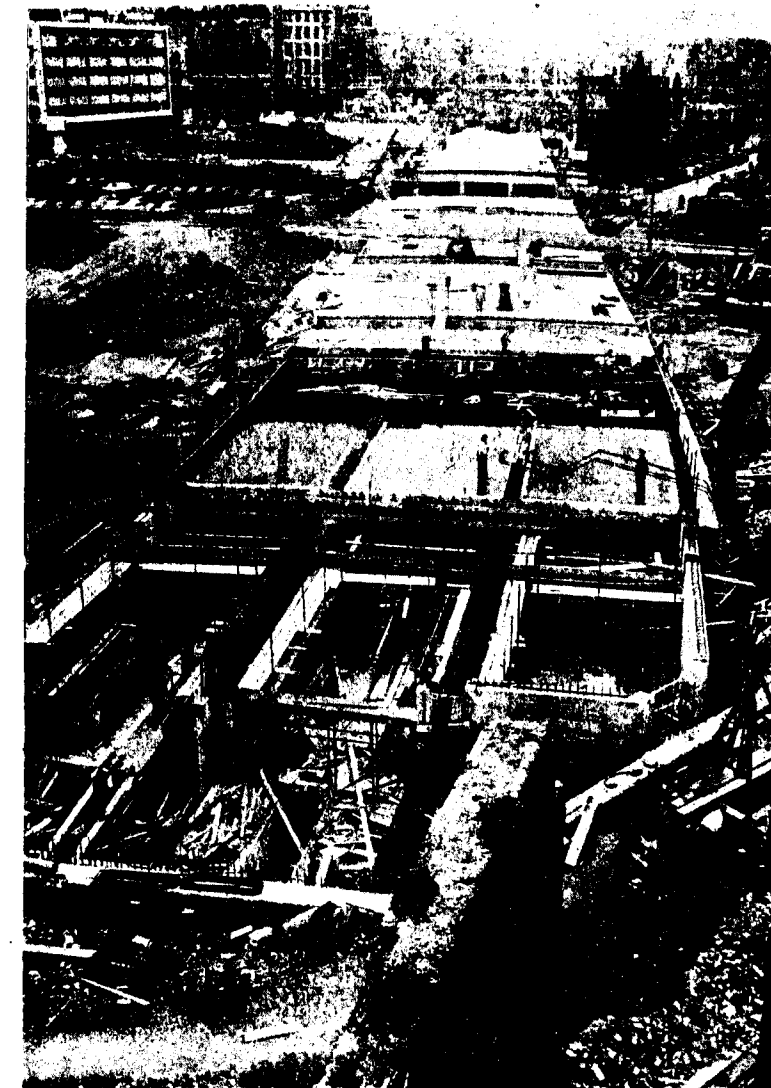
A new trunk road is being constructed through the heart of the City of London, forging its way over some of the worst bomb blitzed areas. It will be a dual-carriageway with three-line traffic in each direction. Garages for several hundred cars are being built below the road. Not the least part of the cost of many millions of pounds has been that of acquiring the land
