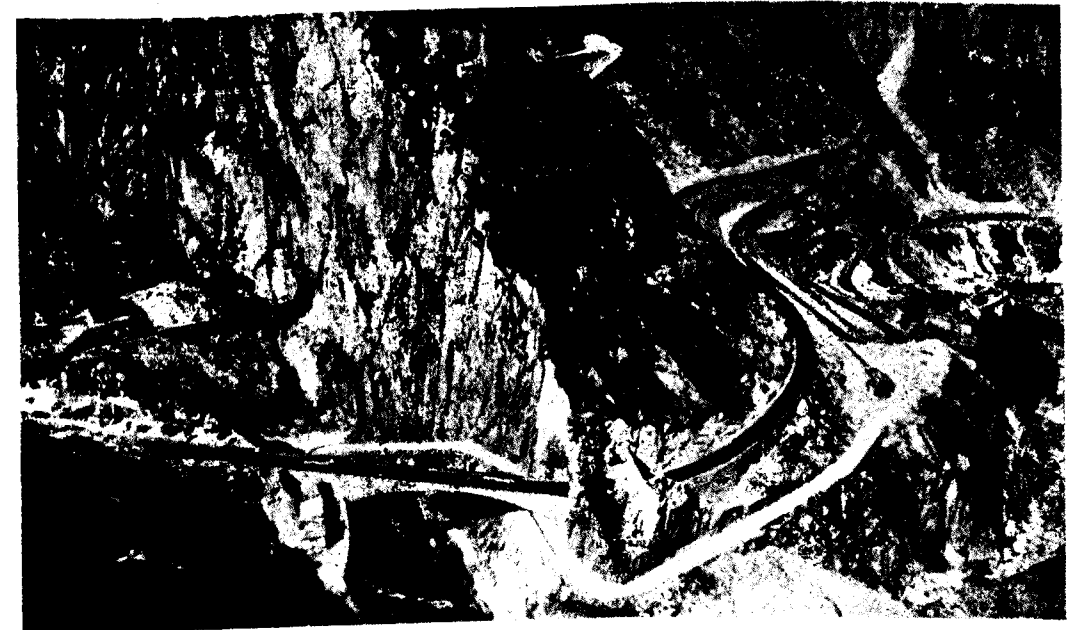
The new road at Schollenen Gorge with the old road below.
