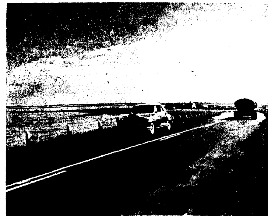
Section of finished pavement along Sask. section T. C. H.
