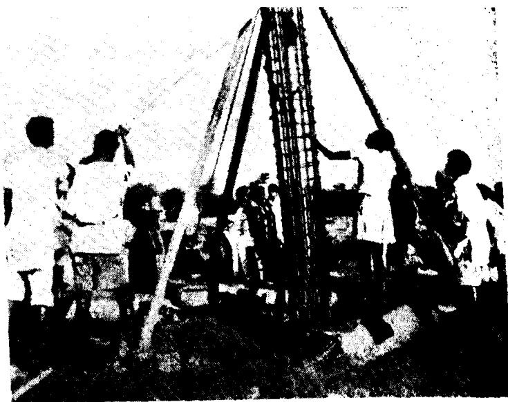
The above view shows work in progress on the construction of 19" diameter Piles For DHAMDACHA Bridge in Naysari Dangs Division for Bombay P.W.D.
