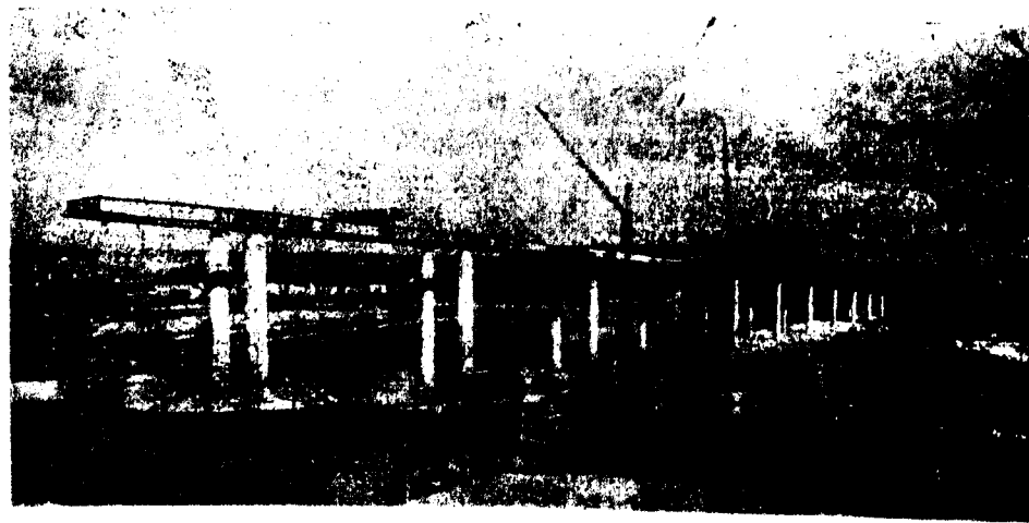
Kettig viaduct under construction, showing the girder support for the formwork, with the device for moving it over the foremost columns.
