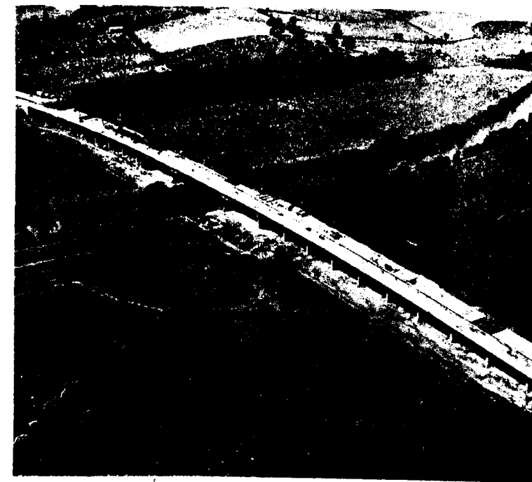
Queenhill Bridge and Viaduct from the south
