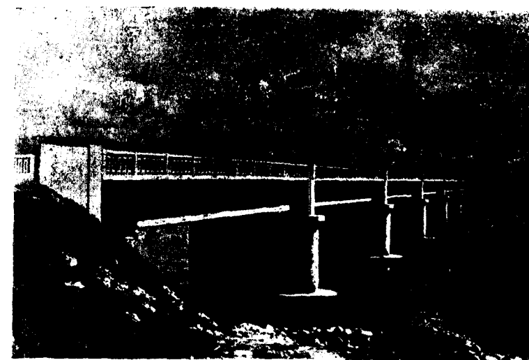
Bridge Over the River Buroi on North Trunk Road In Assam Overall Length—1,056 ft.
