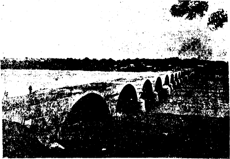
General view of the bridge
