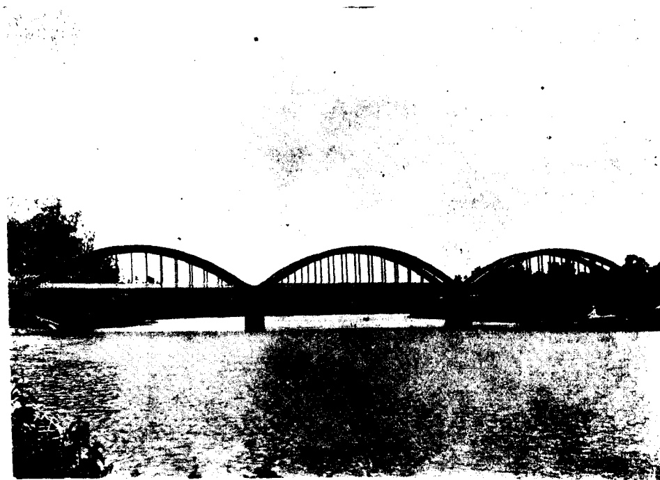
A view of the completed bridge
