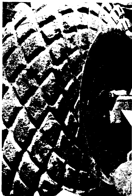
Deterioration caused by oil or grease
