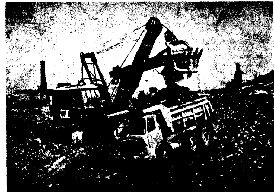
Air-cooled slag for the new automatic processing plant at Port Talbot being loaded for transport to the loading chute leading to the primary crusher
