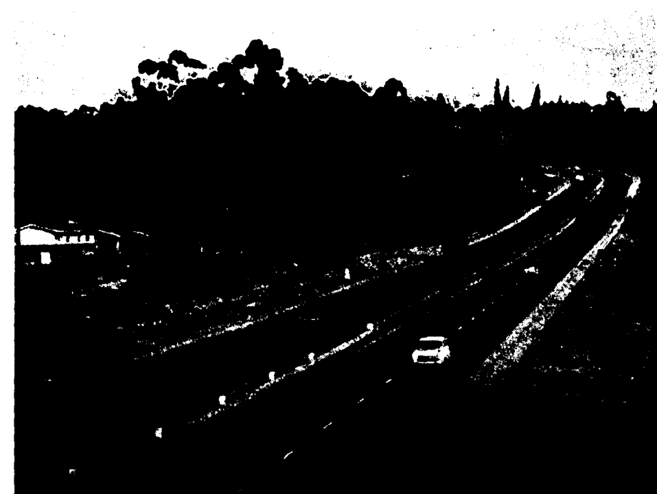
Typical example of dual carriageway construction
