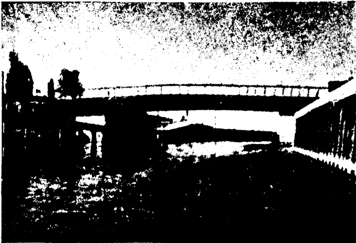
"Hogebrug"—a road bridge over the River Yser at Dixmude. Twelve Preflex beams, each spanning 70 ft, give an overall width of 61 ft, the total construction depth being 2 ft 8 in.
