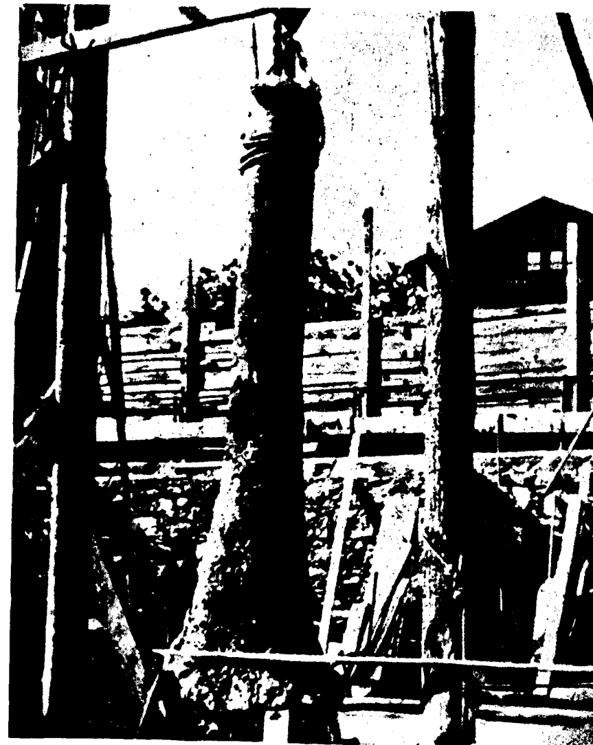
A demonstration pile which has been dug out after driving. This shows completed shank with bulb at base (unreinforced pile).
