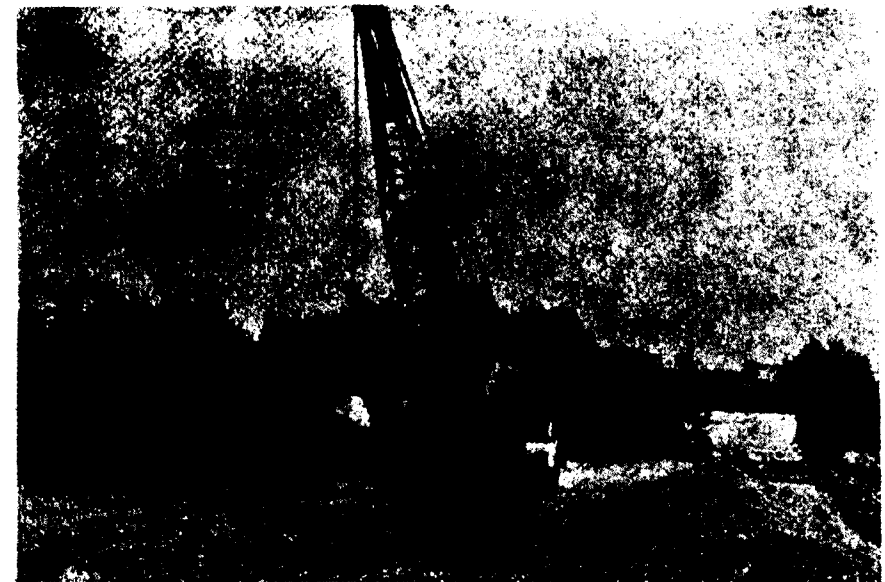
Demolition of old concrete pavement by a 1½-ton steel drop ball, suspended from P & H truck crane
