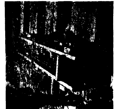
Showing the end blocks in form ready for casting
