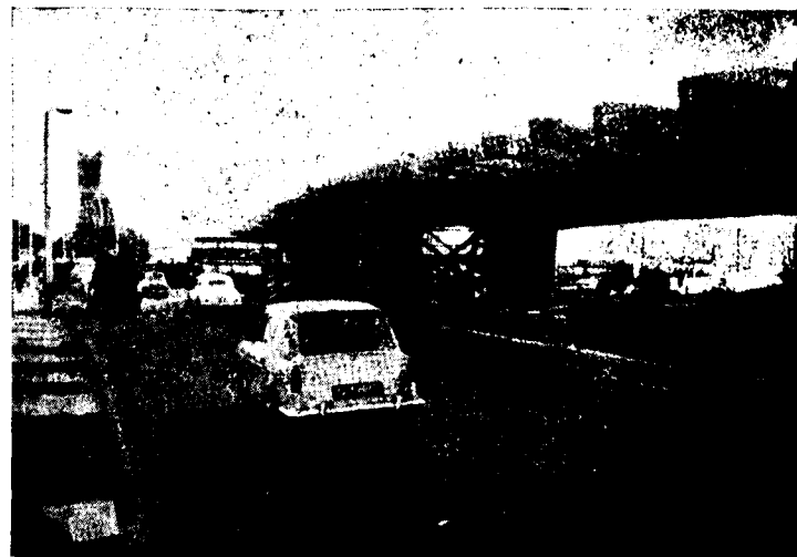
A view of western end of the flyover showing the attractive curve of the continuous hollow spine beam
