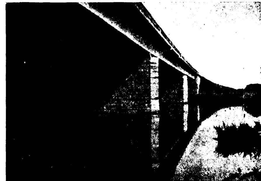
A modern bridge of huge dimension on an autobahn in the State of Westphalia
