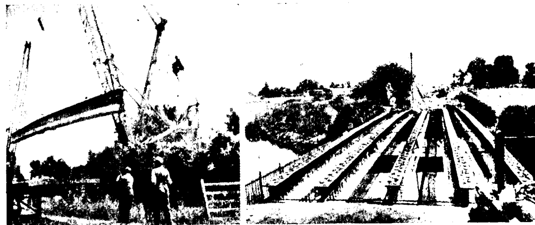
Lowering one of the Preflex beams for the Chippenham Bridge
