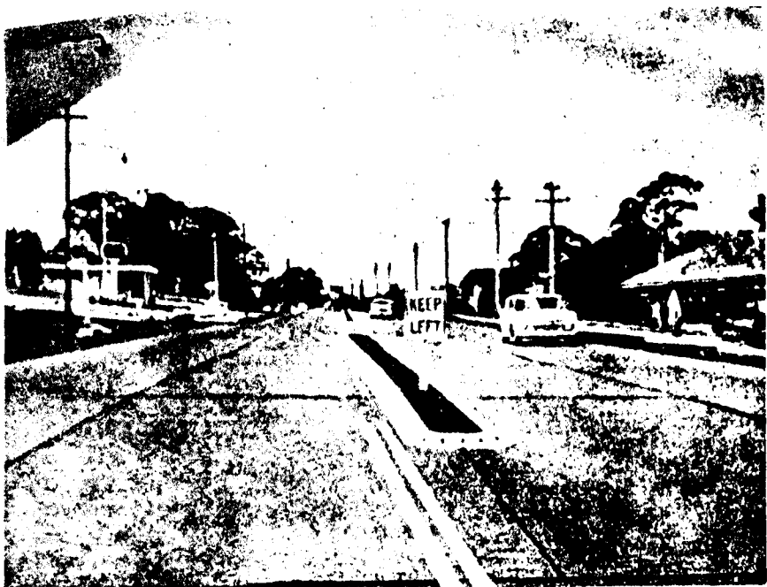
Commencement of a narrow median, showing line marking and sign board
