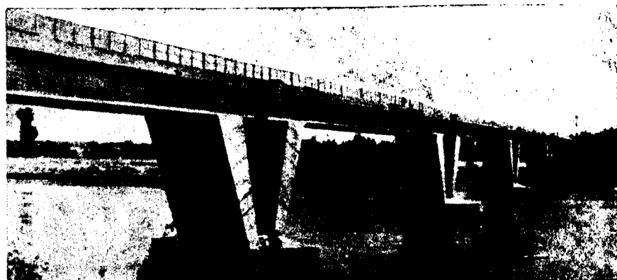
This railroad bridge at La Voulte-sur-Rhone was constructed by cantilevering the concrete in conjunction with prestressed struts, the sliding forms being supported on temporary steel girders. Courtesy S.N.C.F. and Enterprises Boussiren
