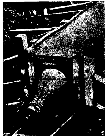
Mountainside culverts in Switzerland are built using deflatable duct-tubes
