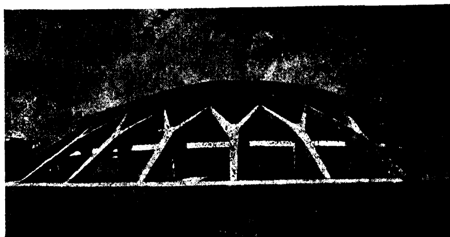
The smaller Palazzetto dello Sport in Rome, also by Pier Luigi Nervi, with Annibale Vitellozzi as architect, has an unusual arrangement of supporting arches
