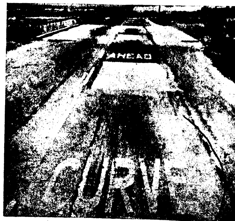
A view of the rock-and-plastic rumble strips constructed in Contra Costa County, Calif., to warn and slow down vehicles approaching the sharp curve in background.
