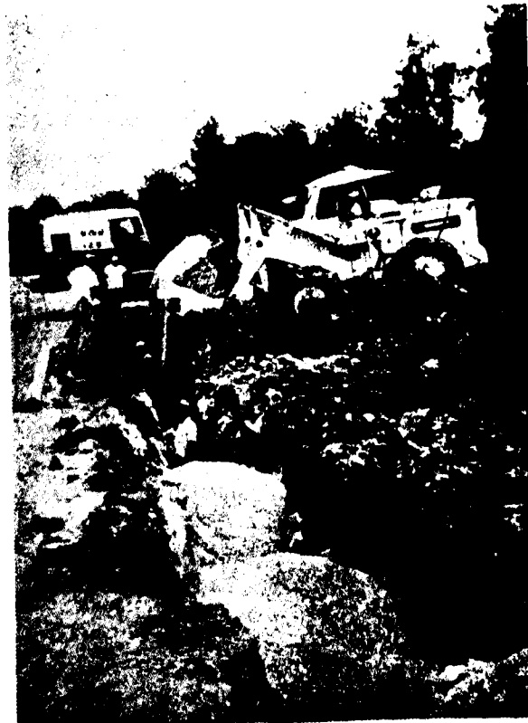
A shoulder drain being installed along a section of finished grade on the North Carolina project here described.
