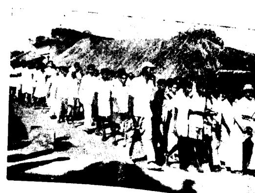
Road completed! Now back to College!
