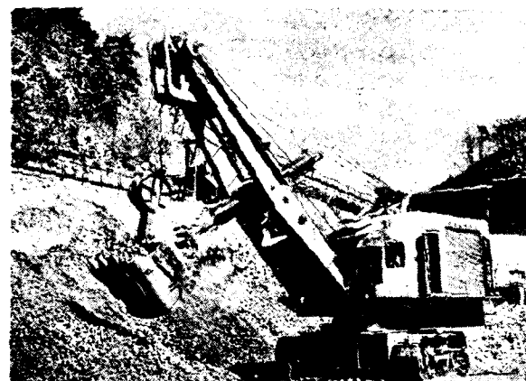
Giant shovel excavator, type E 25, electrically driven
