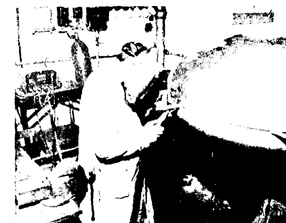
Welding a "14 gauge" Copper bowl with direct current and a Seirion to initiate and maintain the T. I. G. arc.
