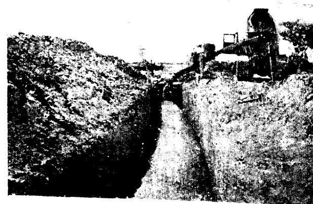
General view showing construction of 48-inch No-Joint Concrete Pipe on curve—Swanston Estates Residential Tract, Sacramento
