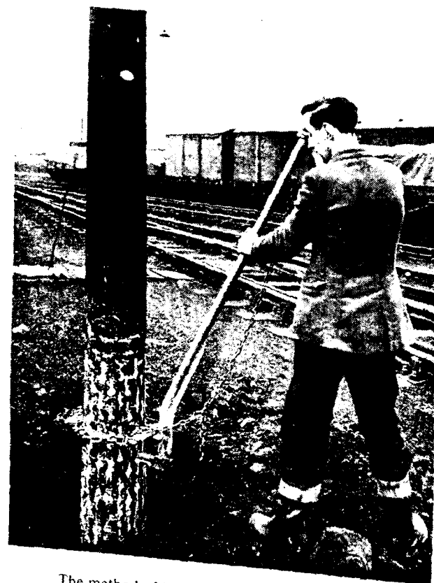
The method of injecting salts into erected poles
