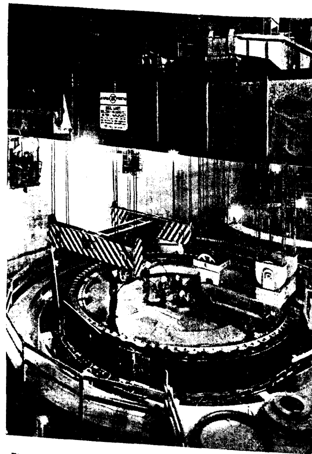
Fig. 6. The 445-ton rotor being lowered into the stator with the aid of two coupled overhead cranes and a yoke. The alignment of the rotor hub after reaching the upper edge of the generator shaft must be extremely accurate both in relation of the shaft and vertically. When the rotor is 300 mm (11.8 in.) from its final position on the shaft, the diameter of the rotor hub is only 0.1 mm (0.004 in.) greater than that of the shaft. (52197. Photographed by Ekholm)
