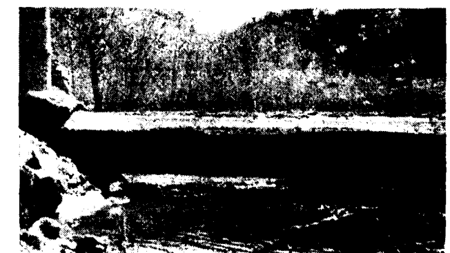
View of 30-inch Dia. No-Joint Concrete pipe suspended over washout. Pipe is suspended for a length of about 45-feet. Soil was eroded during floods of December 1955—on ranch near Westley, California. Pipe was constructed in Aug. 1952. This photo was taken in March 1956.
