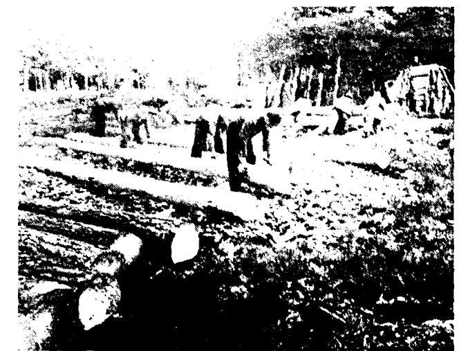
The Diffusion Process. Freshly felled trunks being debarked, treated with Cobra preservative salts and stacked at the felling site.
