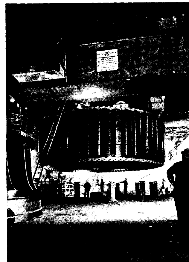
Fig. 4. The complete rotor is raised from its site of erection in order to be moved to the generator pit and lowered into the stator. To the left of the illustration, part of one of the turbine runners can be seen. (52192. Photographed by Ekholtz)
