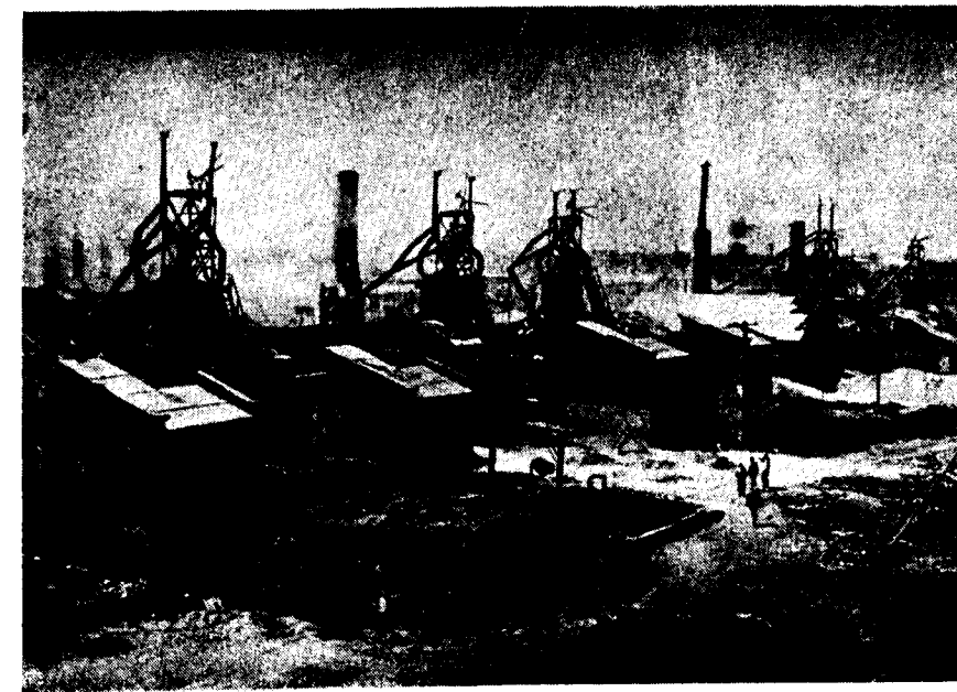
The site of this thriving Hsuanwu Steel Plant was a reed ground more than two years ago.
