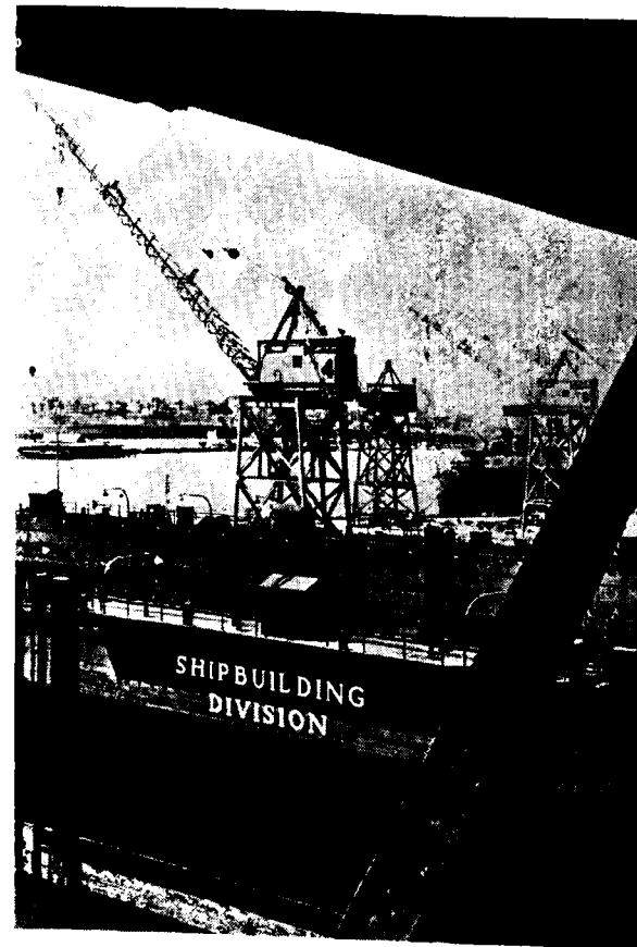
Partial view of the recently enlarged and modernized Los Angeles Harbour Shipyard of Bethlehem Steel Company. In foreground is 15,000-ton sectional drydock; beyond are four of eight huge gantry cranes used in yard's repair and conversion work.
