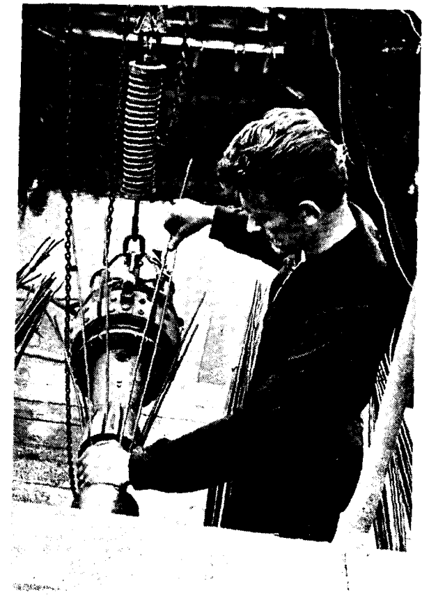
Fig. 6. Anchors for tendons for various prestressing forces ranging from 8 to 100 tons.
