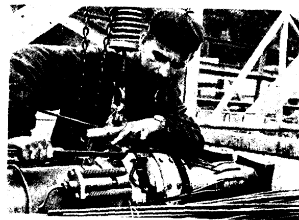
Fig. 3. Clamping of the Wires in the clamping jaws.
