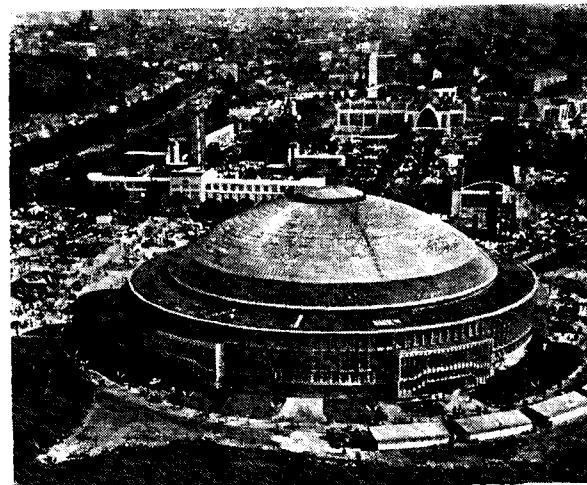
International Trade Fair in Brno.—Pavilion Z built in 1959 ranks among the most impressive buildings on the Trade Fair grounds. It is 38.5 m high and its total area of 18,000 sq. m. is covered by a daring dome of steel tubes laid with a roof of aluminium sheet, glass and plastics.
