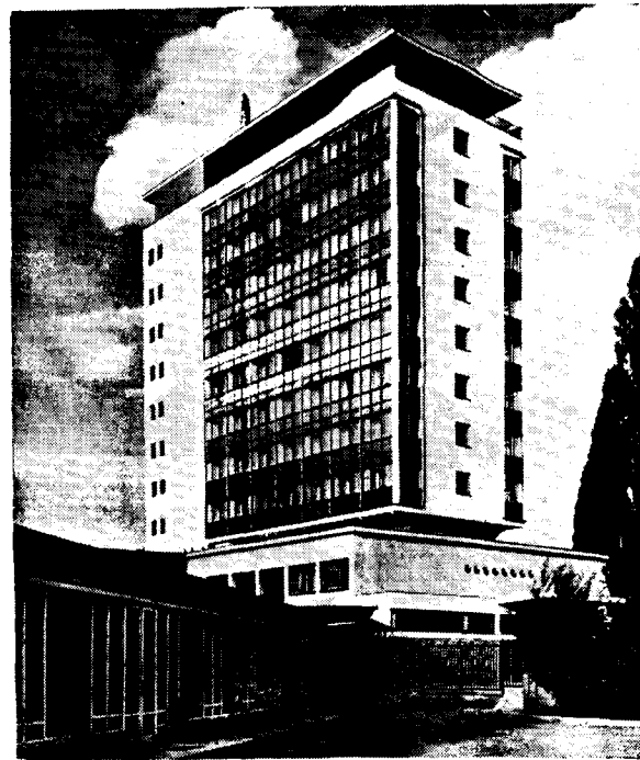
International Trade Fair in Brno—The administrative building, the commercial centre during the time of the Trade Fair, where representatives from all over the world meet to discuss business.
