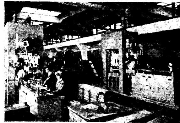
Automatic presses for the pressing of stationary and rotor part plates.
