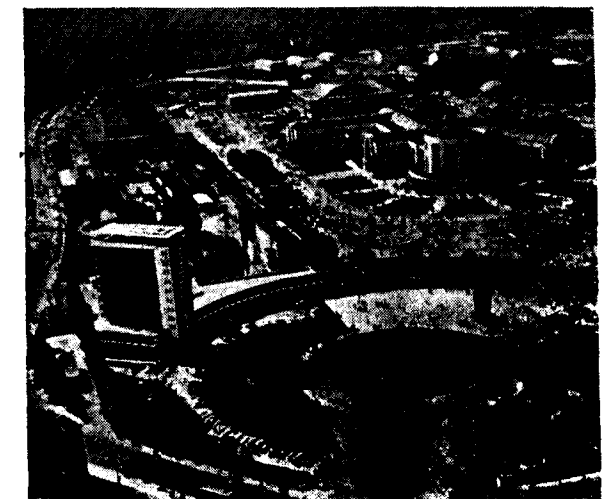
International Trade Fair in Brno.—Aerial view of a part of the Trade Fair area showing the multi-storey administrative building.
