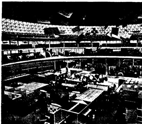
International Trade Fair in Brno.—Interior view of pavilion Z, the total area of which is 18,000 sq. m. The pavilion was built in 1959; its modern circular ferro-concrete construction has attracted the admiration of experts from all over the world.
