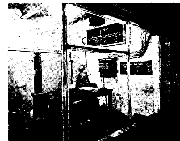
Train despatcher's cabin for routing outgoing trains of empty trucks
