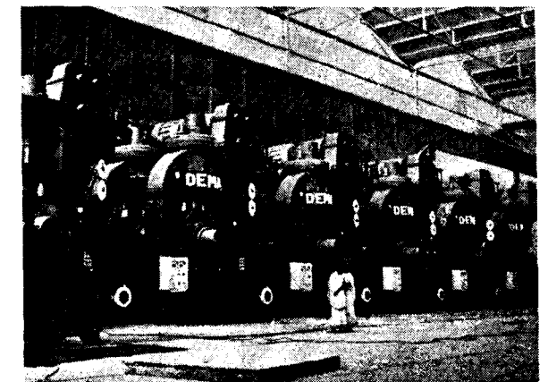
With the official inauguration of the Wide Strip Mill the last of the large-scale plant at the Rourkela iron and steelworks is now complete. This mill will produce wide strips which India so urgently needs. Annual capacity is 1 million tons. The Wide Strip Mill consists of two roughing stands and a six-stand finishing mill which is shown on the picture. It is the most modern mill of its kind in the whole of Asia and can be operated by very few personnel. Production is fully automatic.
