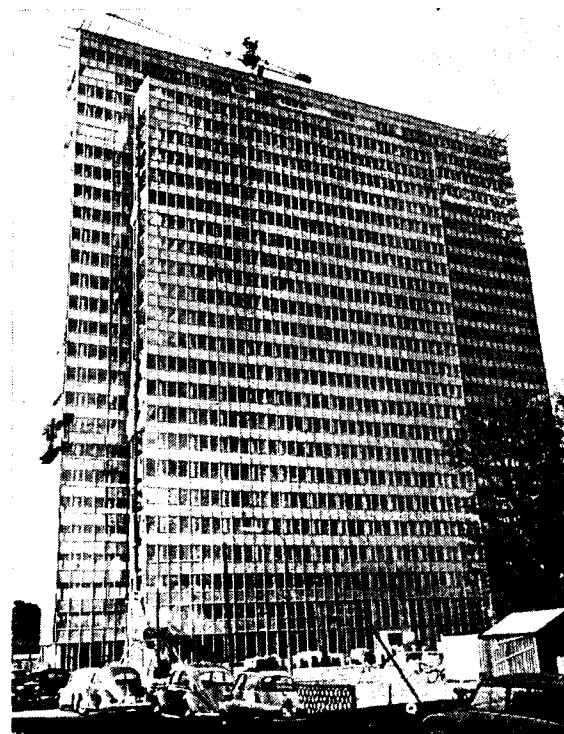
Phoenix-Rheinrohr Skyscraper in Düsseldorf, under construction. The shell walls consist of enamelled steel sheet plates and plate-glass. The plate-glass has the full height of the storey.
