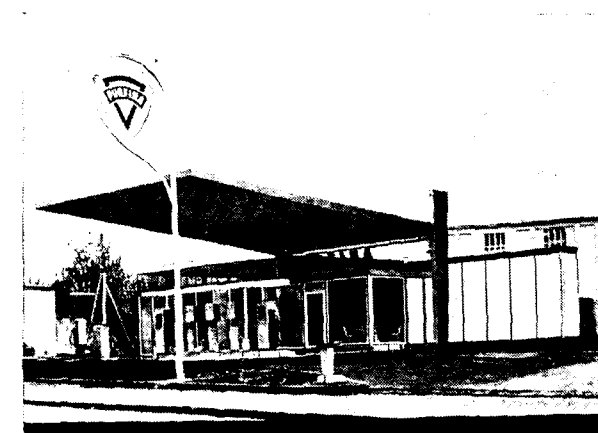
Fina filling station at Frankfurt/Main, consisting of prefabricated wall elements of enamelled steel sheet and roofing of corrugated steel sheet.
