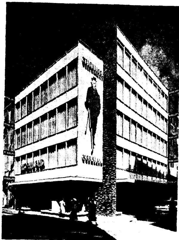
Department store with shell walls of enamelled steel sheet walling plates.
