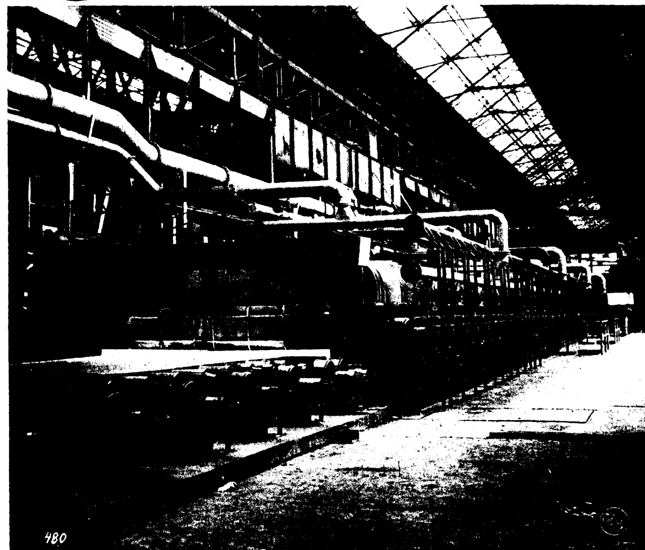
Plate Normalizing Furnace
