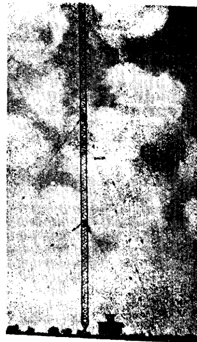
Antenna Tower for a High-Power Transmitter
