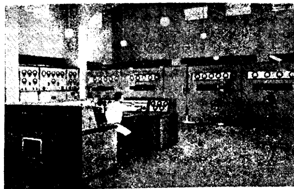
Two 100 kW Short-wave Transmitters, "A" side
