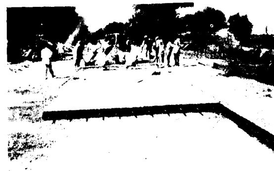
Photo 5 Showing dowel bars at expansion joint
