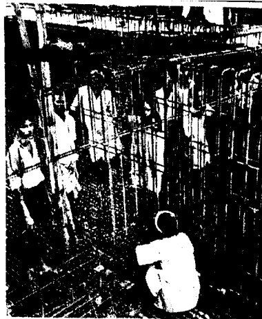
Photo 5. Reinforcement for intermediate diaphragm
