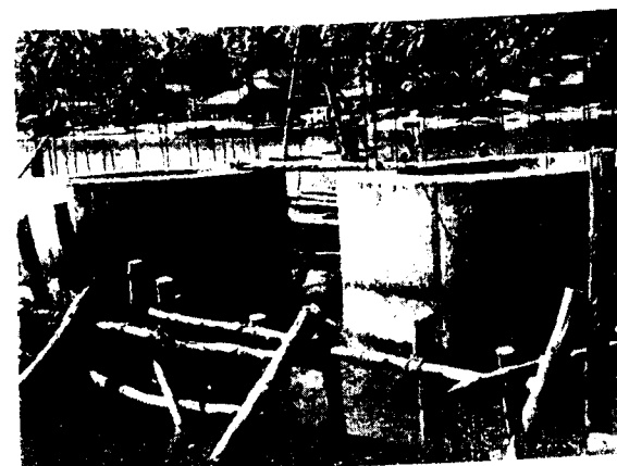
Photo 2 Well ready for sinking
