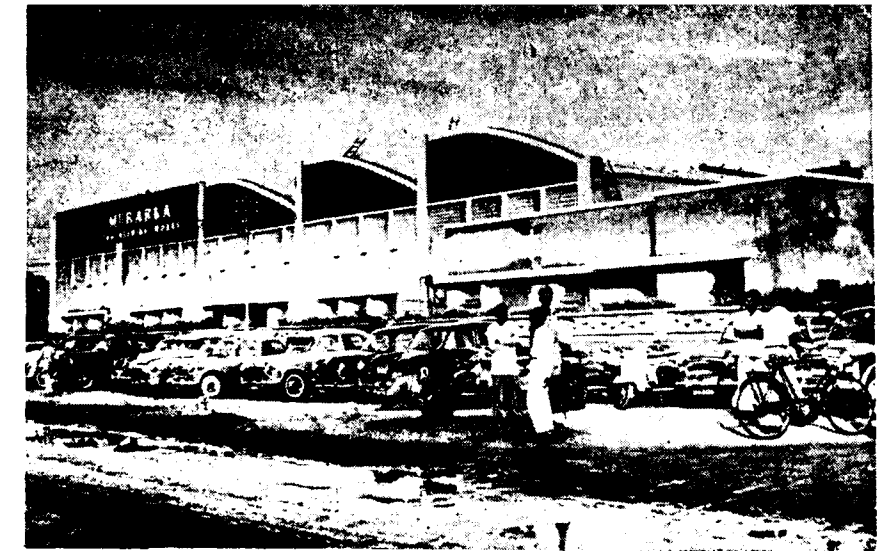
1. Front view of Factory
