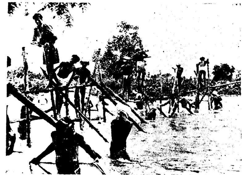
Breaches in Arasalar River on the western side of Kumbakonam Town are being closed by the workers of Raman & Raman (P) Ltd., Kumbakonam. These breaches were mainly responsible for the inundation of Kumbakonam Town.
