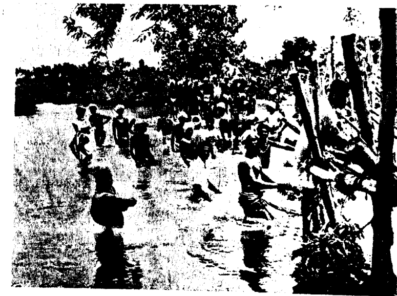
Breaches in Arasalar River near Mangudi (3 miles West of Kumbakonam) Closing of breaches in progress.
