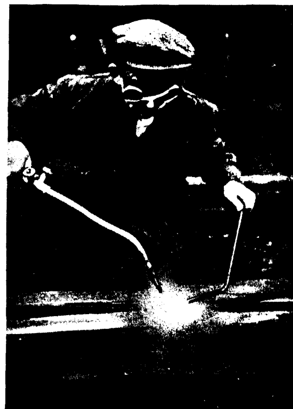
Action Picture of a Welder Rebuilding Worn Rail Track.
