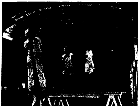
The interior surface of the coach is sprayed with asbestos to make it heat and sound proof.
