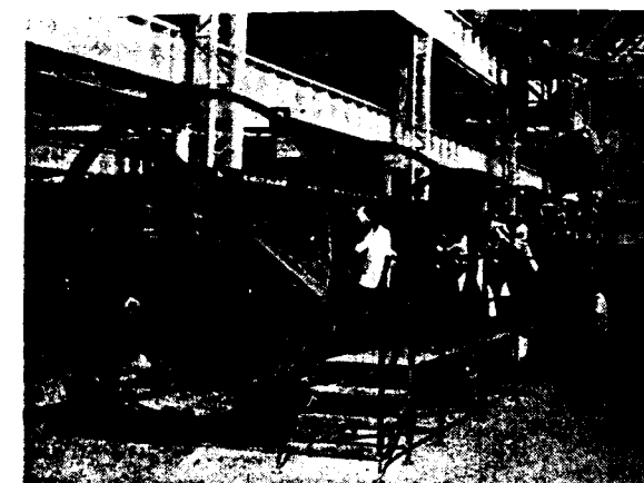
All components are then fed into the Main Assembly Shop where roof is assembled in the roof jig
