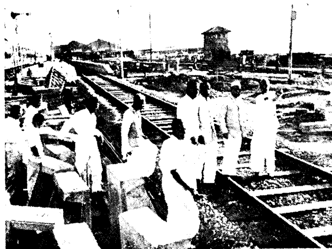
Remodelling Madras Central Station : Railway Deputy Minister inspecting the progress
