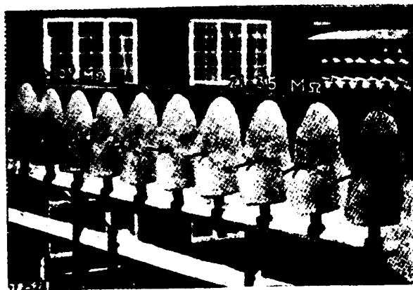
Fig. 2. Telephone insulators covered with snow. Spring 1954.
