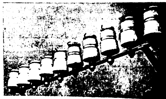
Fig. 3. New telephone insulators after two years' service.
